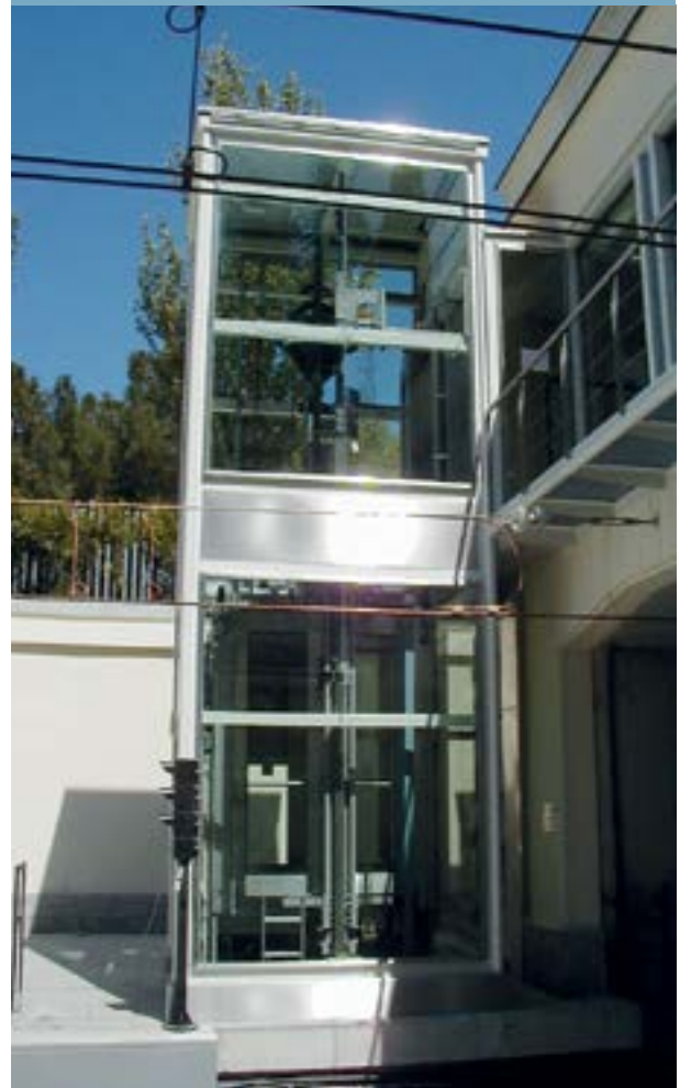
Figure 3. Self-standing steel shaft
